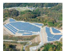
Mega-solar power business
